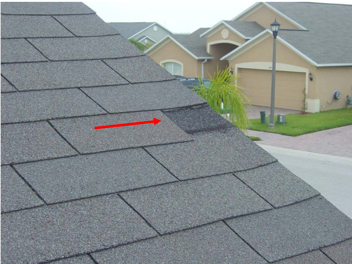
Missing shingles
