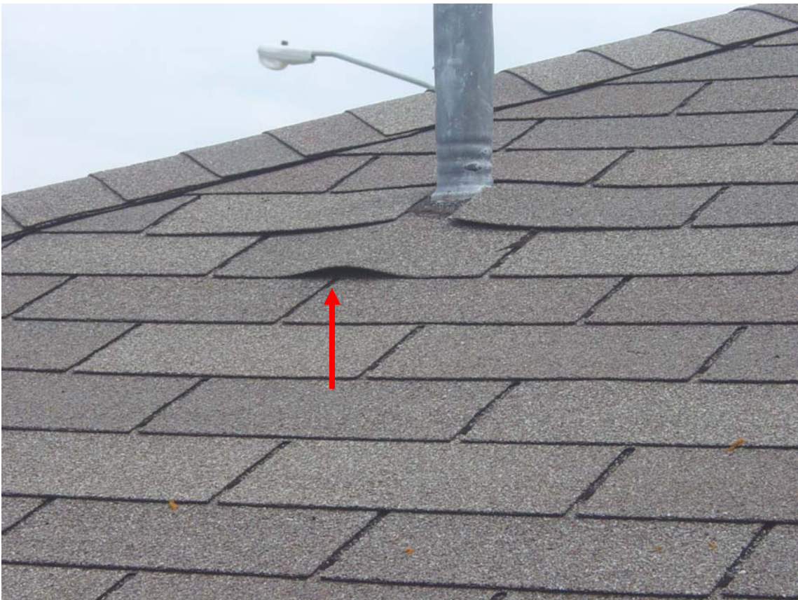
Lifting shingles
